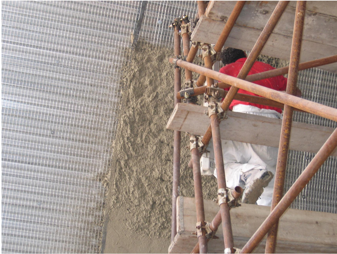
Spray Installation of FireBarrier 135 onto mesh installed onto the corrugated steel cladding (video is available on request)
