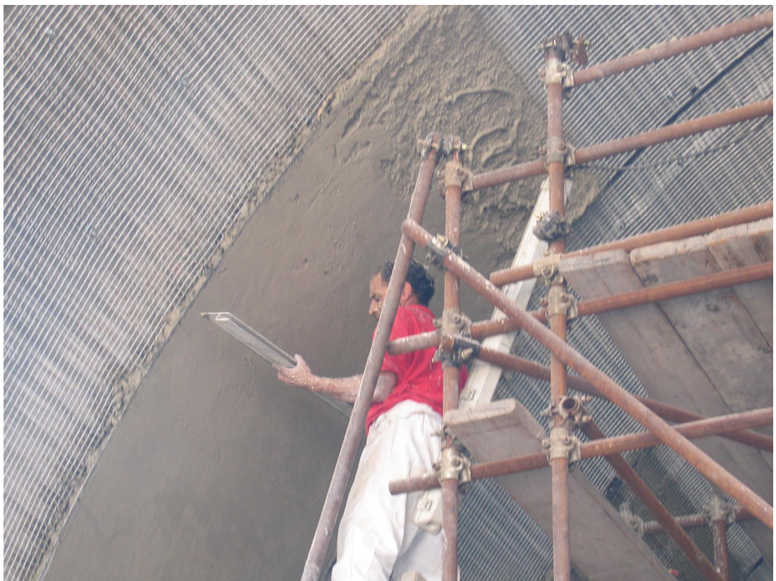
Spray Installation of FireBarrier 135 onto mesh installed onto the corrugated steel cladding (video is available on request)
