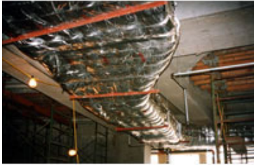
Zero clearance to combustibles
